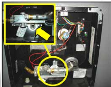
Water Heater Drain Plug Location
