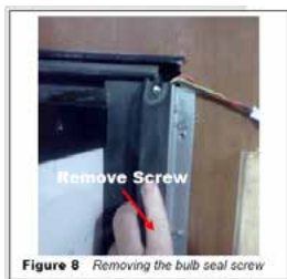
Figure 8 Removing the bulb seal screw
