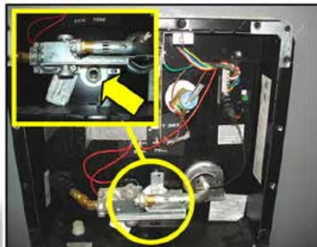
Water Heater Drain Plug Location
