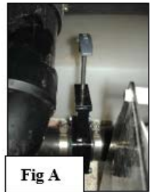
Macerator Cutoff Normal Position
