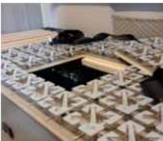
Water heater Bypass Access
