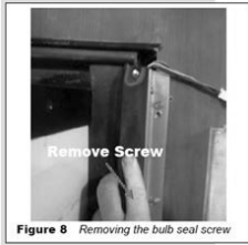
Figure 8 Removing the bulb seal screw
