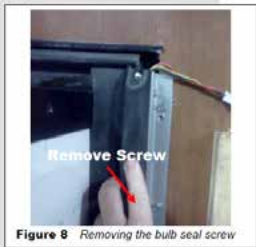
Figure 8 Removing the bulb seal screw
