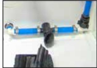
Water supply shutoff to the cartridge water filter (shown OFF)
