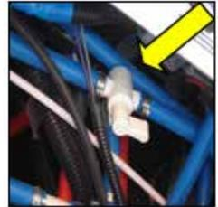
Water supply shutoff to the canister water filter shown ON
