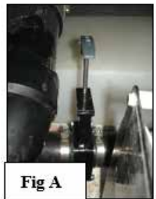
Macerator Cutoff Normal Position
