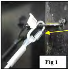
Fig 1 Quick Link cable hook-up at top of the door frame
