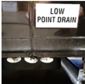
Low Point Drain Example
