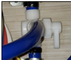
Fresh Water Tank 3 Way Valve Example (If Equipped)
