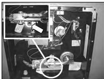
Water heater drain plug location
